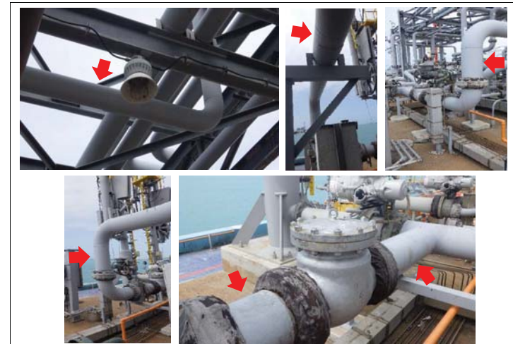
Photo6: 66HV218 to ballast line still in good condition observed.
