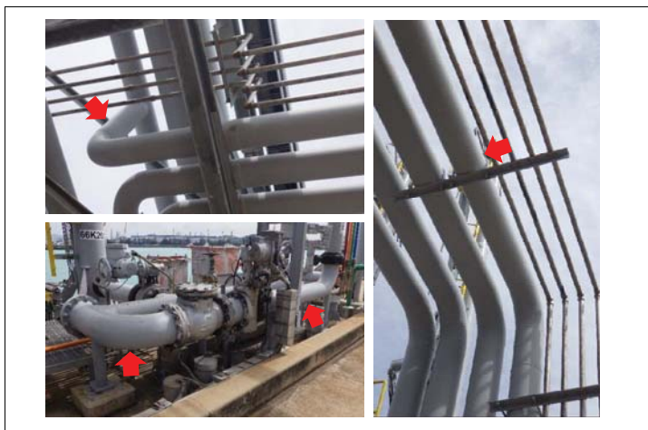
Photo8: 66K203 to ballast line still in good condition observed.
