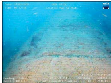
Typical Field Joint
