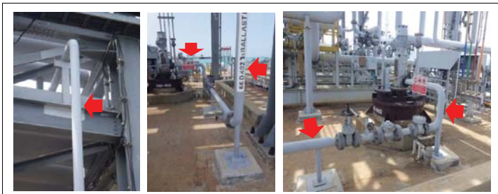
Photo12: 66D402 to ballast line still in good condition observed.
