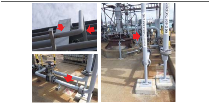
Photo13: 66D401 to ballast line still in good condition observed.
