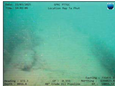
Typical Field Joint
