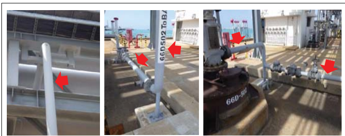
Photo14: 66D502 to ballast line still in good condition observed.
