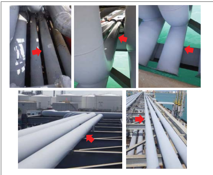
Photo4: Ballast line at shore line to pipe rack still in good condition observed.
